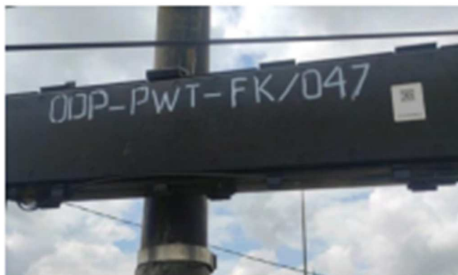
Gambar 2.4 ODP ( Optical Distribution Point )
