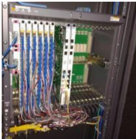
Gambar 2. 5 Optical Line Terminal (OLT) [5]
