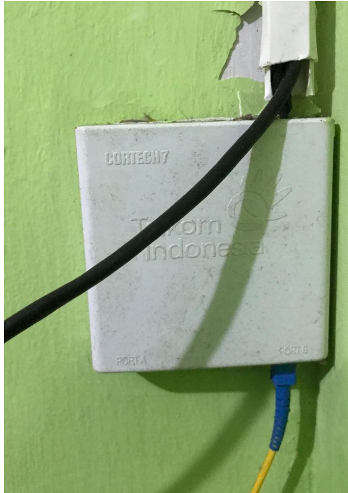
Gambar 2. 9 Optical Termination Premises (OTP)
