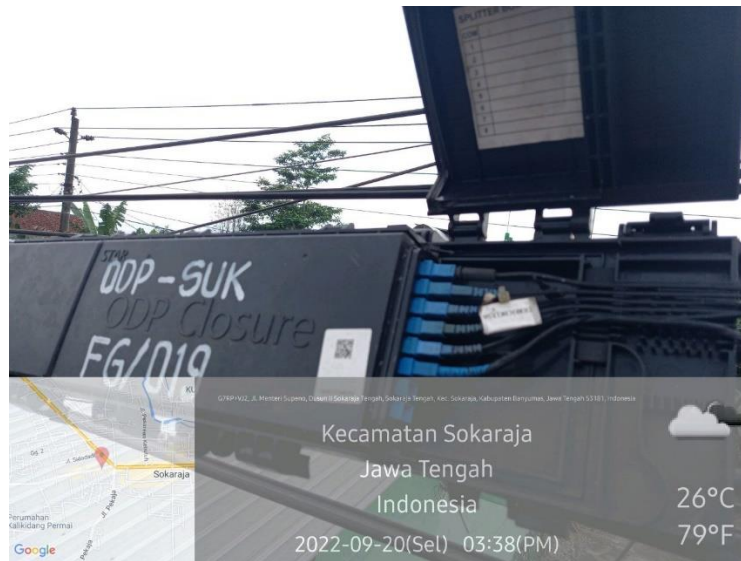
Gambar 2. 7 Optical Distribution Point Closure
