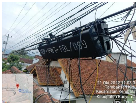
Gambar 2. 5 Optical Distribution Point (ODP) [7]
