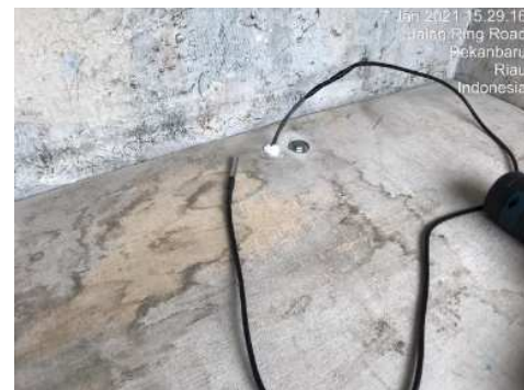
Fig. 5. The installation of temperature sensor in motorcycles
