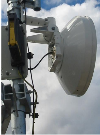
Gambar 2.2.2 Antena Microwave
