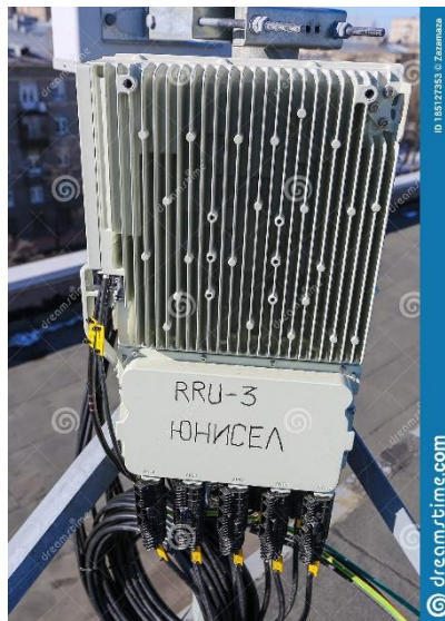
Gambar 2.2.3 RRU ( Radio Remote Unit )
