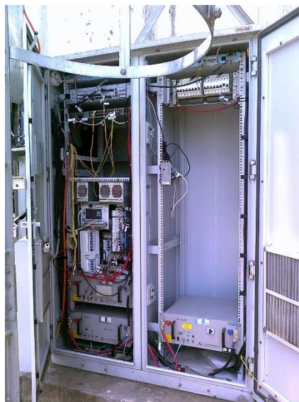
Gambar 2.2.4 Base Transceiver Station (BTS)
