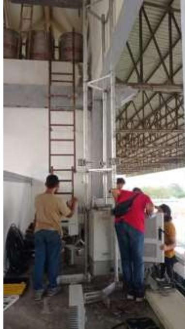
Gambar 3. 3 Proses membangun Combeth BTS
