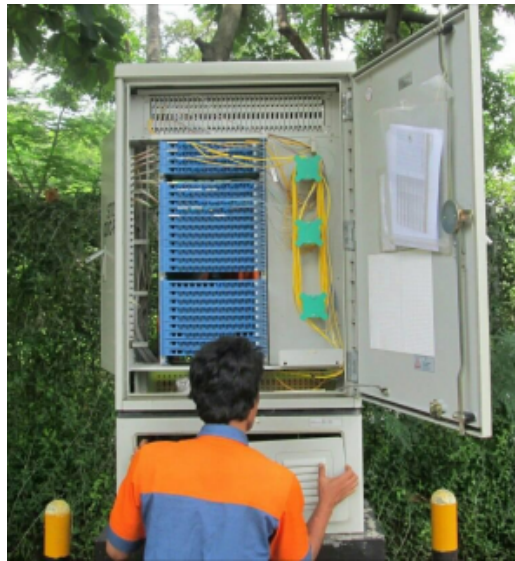
Gambar 2.4 ODC ( Optical Distribution Cabinet )
