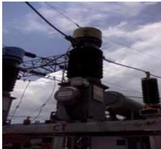
Gambar 2.2 Current Transformer [1]
