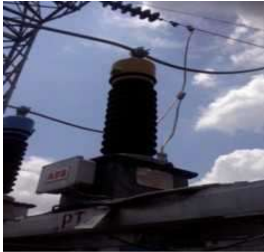
Gambar 2.3 Potensial Transformator [1]
