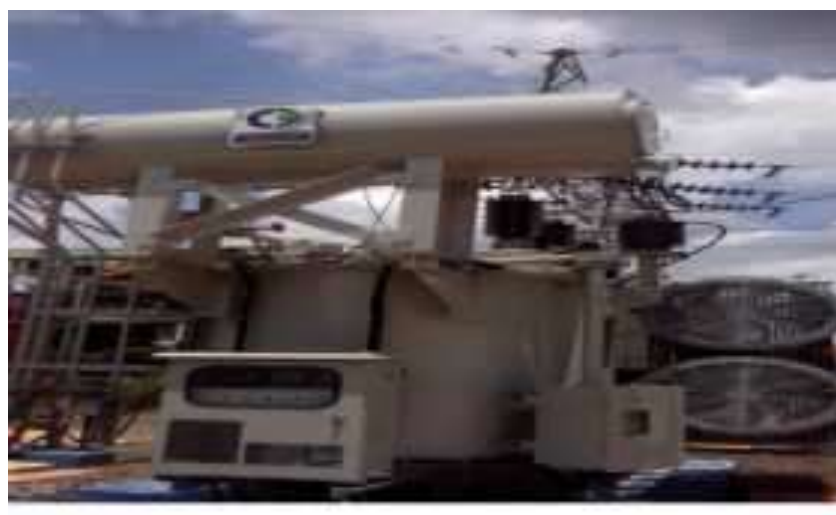
Gambar 2.4 Transformator daya [1]
