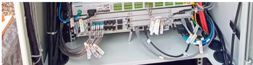
Gambar 2.9 BBU ( Base Band Unit )
