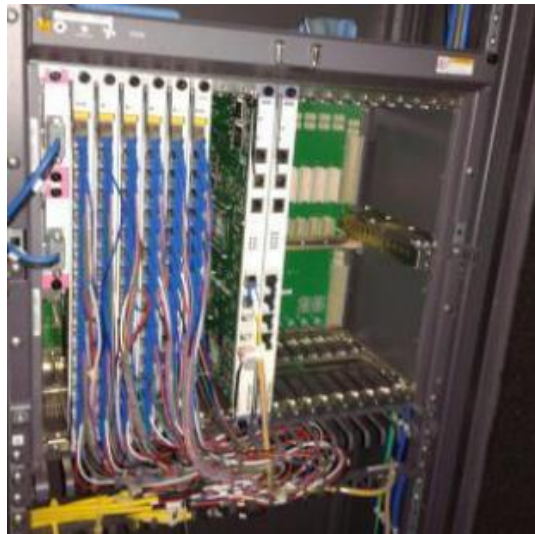
Gambar 2.2 Optical Line Terminal (OLT) [11]
