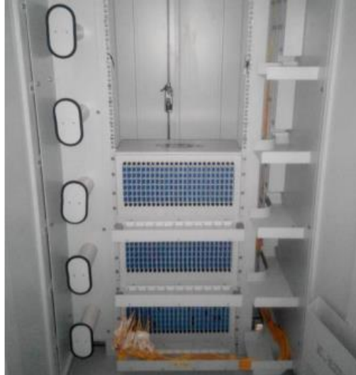
Gambar 2.3 Optical Distribution Frame (ODF) [11]
