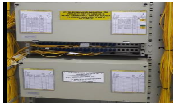
Gambar 3.2 Optical termination Box (OTB)
