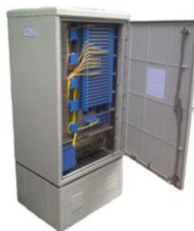
Gambar 2.10 ODC ( Optical Distribution Cabinet )
