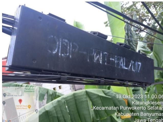
Gambar 2. 2 ODP (*Optical Distribution Point*)
