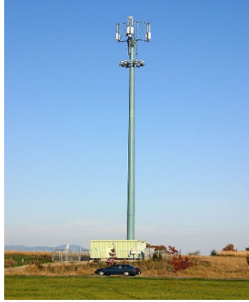
Gambar 2.3 Model menara monopole GREENFIELD [8].
