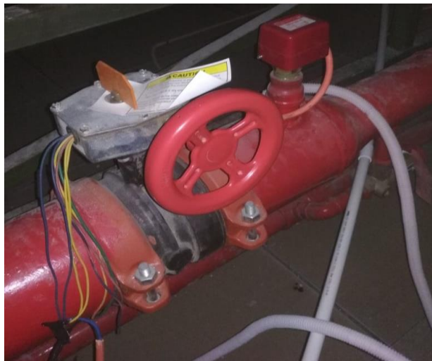
Gambar 2.4 Tamper Switch
