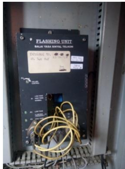
Gambar 8 Rangkaian Flashng Unit
